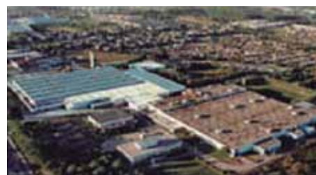
Centro Industrial Córdoba
